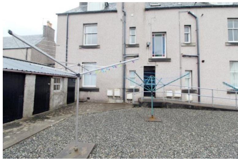
Rear Aspect & Drying Area
