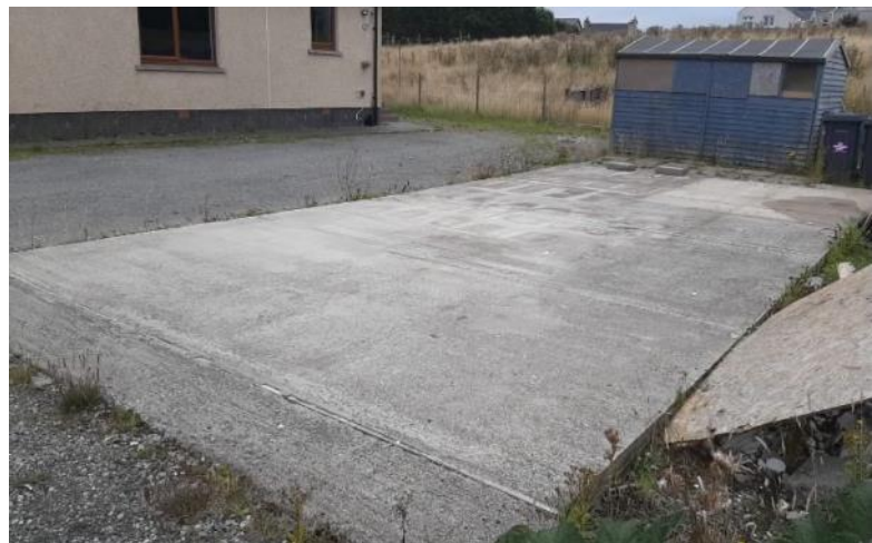
Concrete base for garage/building
